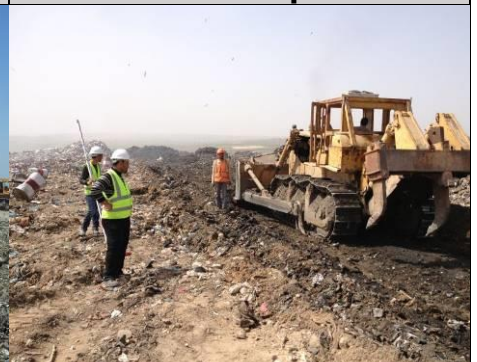
Levelling works in Johr Al Dik
