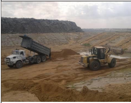
Levelling of hazardous waste cell
