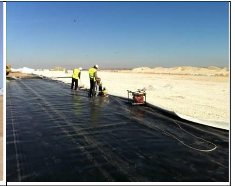
Installation of PE and Geotextile
