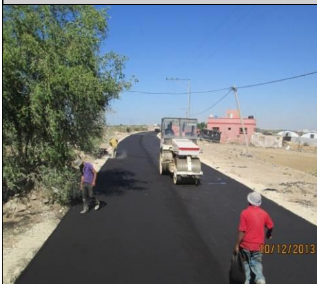
Asphalt for landfill road
