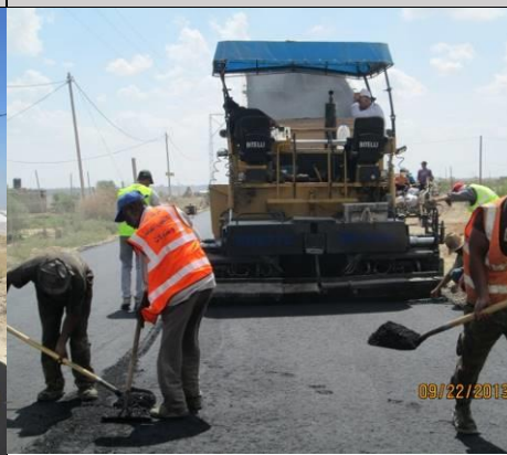
Asphalt for landfill road
