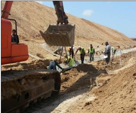
Construction of water channel Landfill
