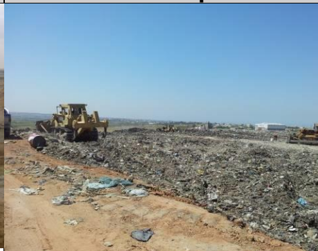
Levelling works in Johr Al Dik
